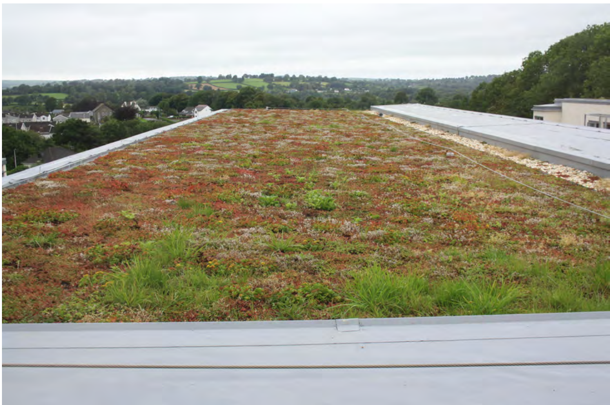
Picture 5.4 Living Roof (Copyright Chris Jones)
